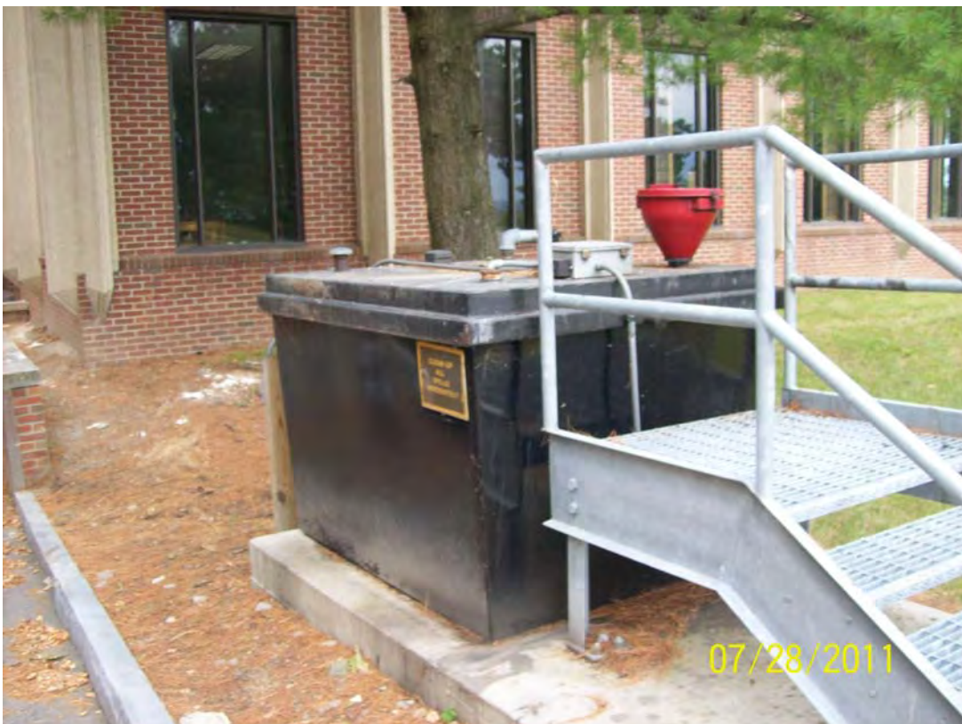
Photo 8: Photo of one of the four waste kitchen grease containers. Each of the four containers are of similar design. Two are 300 gallons in capacity and two are 500 gallons in capacity.
