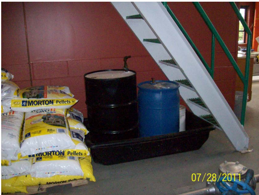
Photo 6: Photo of the drum storage area located in the heating plant.
