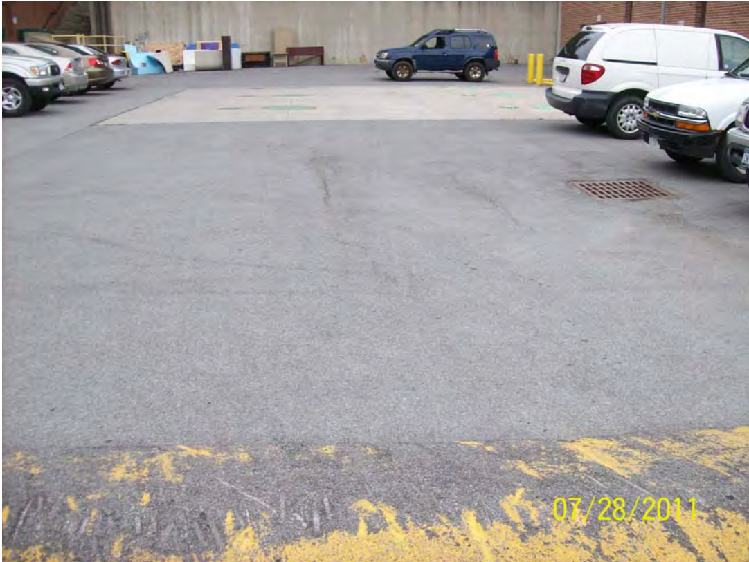
Photo 5. View of the unloading area associated with three USTs (PBS Tank #s 016, 017 and 018). Catch basin visible in picture directs flow to an oil water separator.
