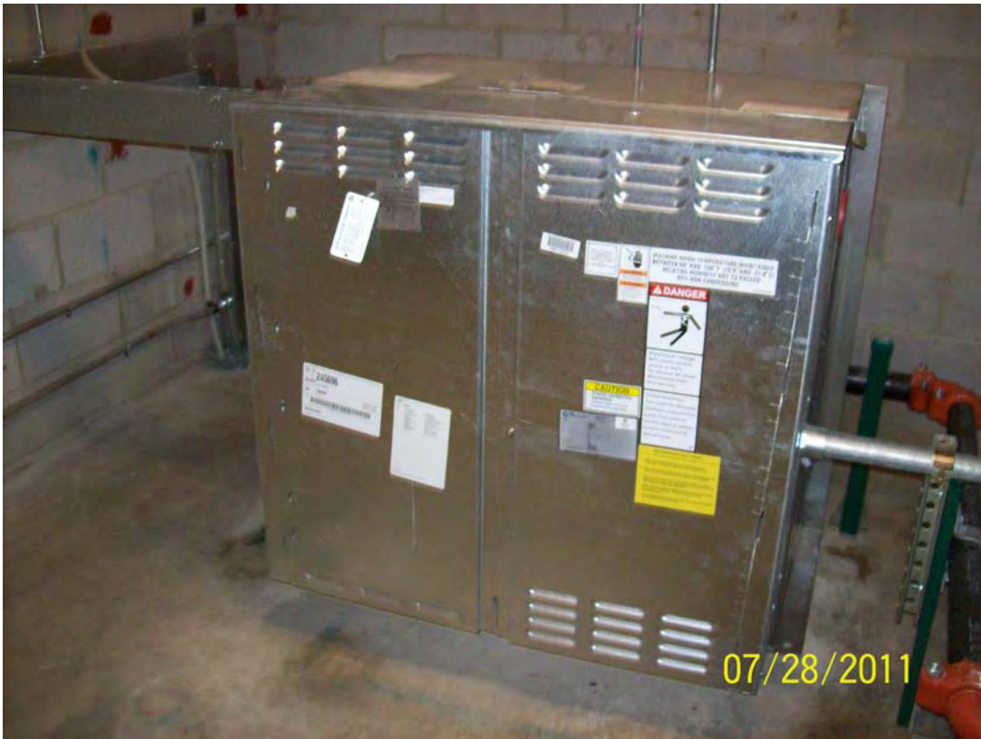
Photo 9: Photo of one of the elevator reservoirs maintained at the facility.
