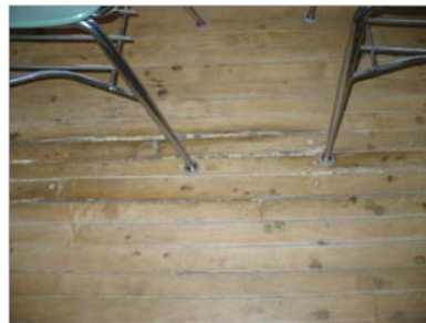
Wood flooring in the classrooms is in poor condition.
