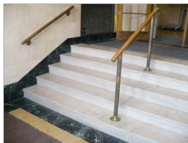
Handrails do not meet requirements of the accessibility guidelines.
