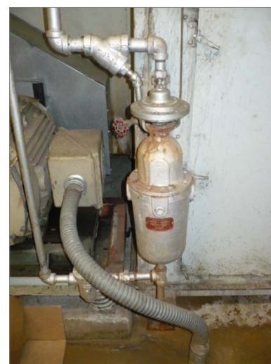
Typical direct injection steam humidifier
