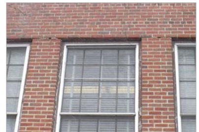
Mortar at the head of the windows is beginning to deteriorate.
