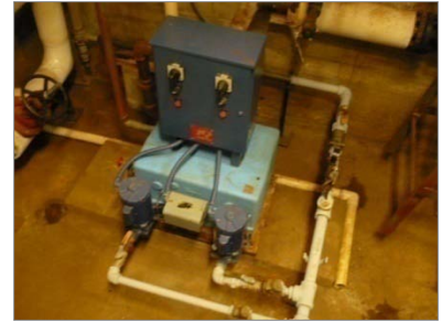
Main condensate pump/tank set
