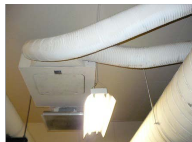
Pneumatic control air compressor
