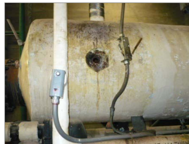
Abandoned steam hot water tank
