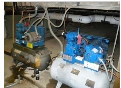
Pneumatic control air compressors
