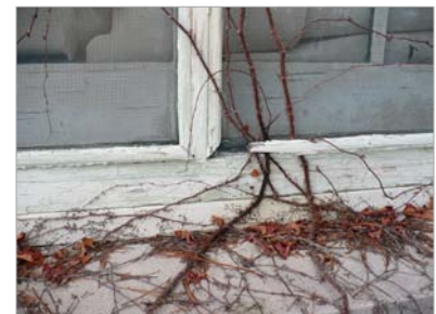
Windows are in poor condition and should be replaced with energy efficient units.
