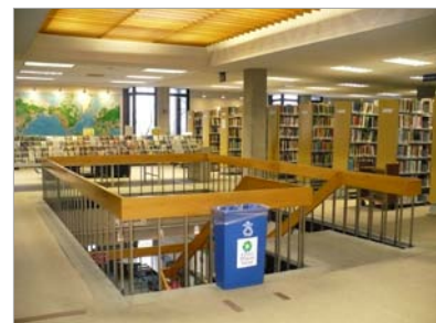
Handrails are not accessible and do not meet requirements of the New York State Building Code.
