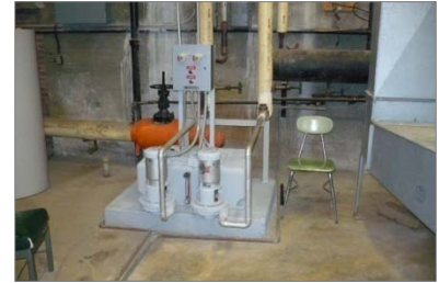
Main condensate pump/tank set
