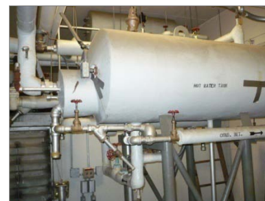
Steam-water storage hot water heater
