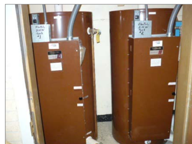
Electric water heaters
