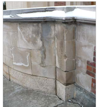
Retaining walls around the perimeter of the building are in poor condition.
