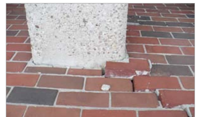
Brick paving around the perimeter should be replaced.
