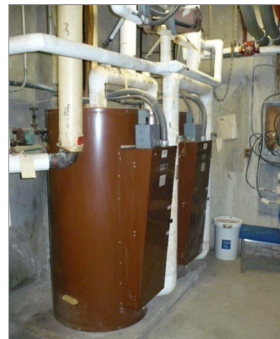
Electric water heaters
