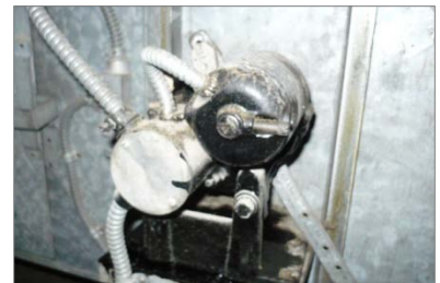
Original damper motor/actuator
