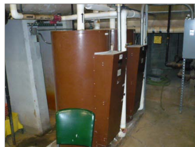
Abandoned steam hot water tank
