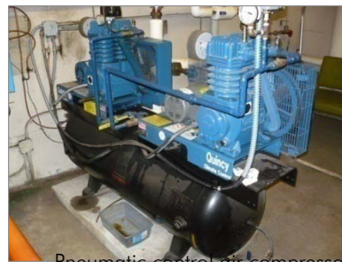
Pneumatic control air compressor
