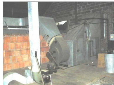
Auditorium supply and exhaust fans
