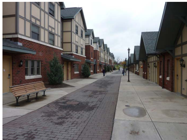
The stamped asphalt at Saratoga Terrace has lost its color and settled in many places, creating low spots and puddles when it rains.
