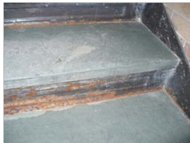
Metal stair risers are rusting.
