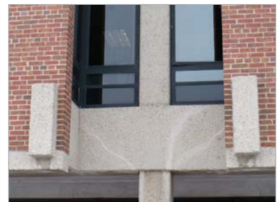
Cracks in the exterior walls indicate building settlement.
