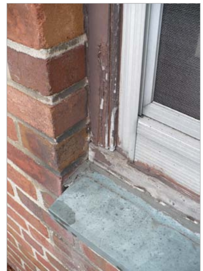
Windows are in poor condition and should be replaced with energy-efficient, double-glazed units.
