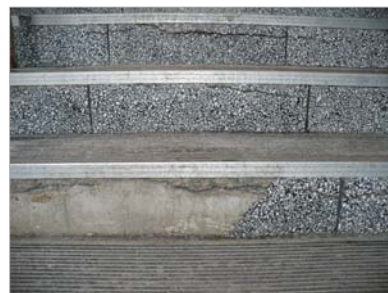
Worn stair treads should be replaced.
