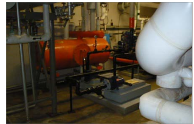
Steam flash tank and return pumps
