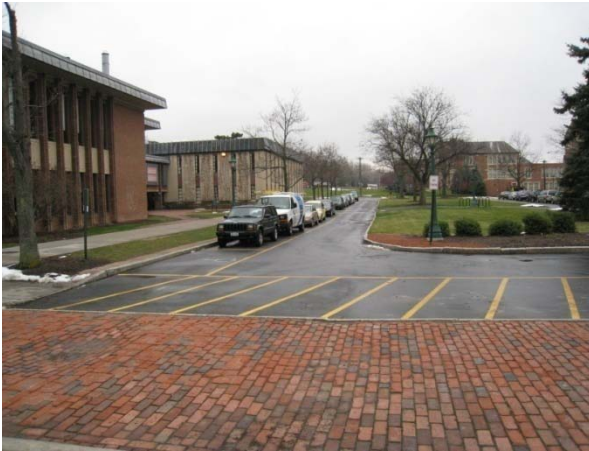
Brick unit pavers, asphalt paving, and granite curb at College Circle are showing wear and tear.
