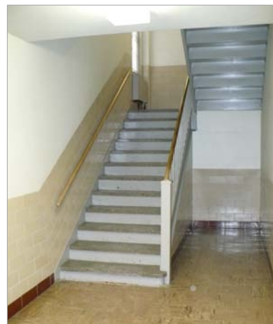
Handrails are not accessible.
