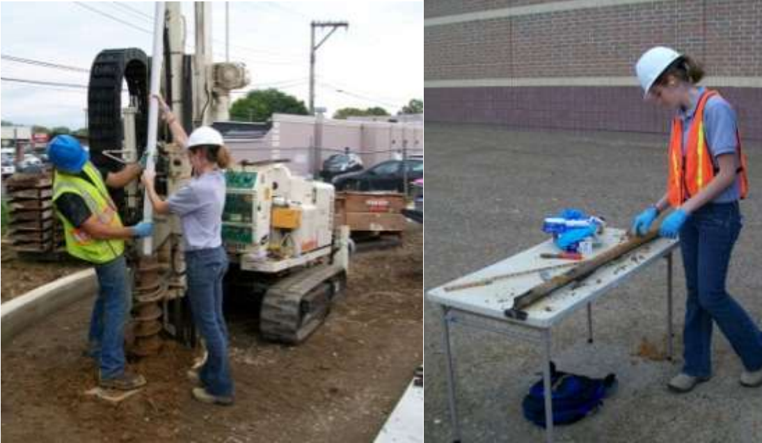
Intern Christa Stell ('13) assisting a driller in the installation of groundwater monitoring well (left) and examining a soil boring to complete a lithographic log (right)
