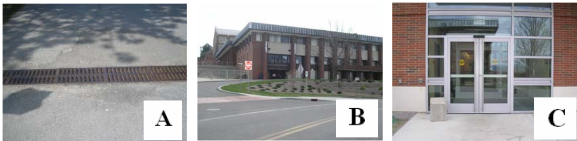
Figure 2. Man-made obstacles. A) This picture was taken next to the Knight Spot. The grate bisects the walkway and is an example of an obstacle as well as a safety concern. Wheel-chair wheels can easily become trapped in the holes. A simple solution would include grates that ran in a horizontal direction. B) This picture was taken on the west side of MacVittie Student Union. Two handicap spots are located at the bottom of the circle and require the person to travel a significantly long distance to enter the Union. Two handicap spots are also located at the top of the circle but are metered. C) This picture was taken at the side-entrance of the Integrated Science Center. A concrete block prevents the door from being opened fully and also prevents access to the push-button door.
